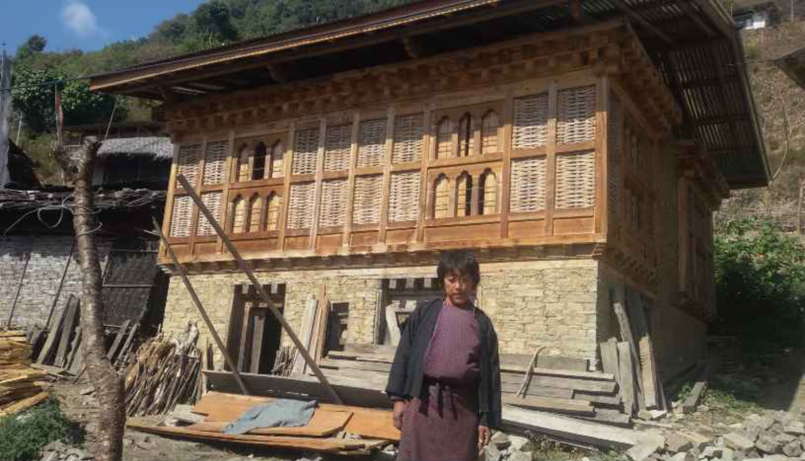
A new house under construction in Wama, Monggar
