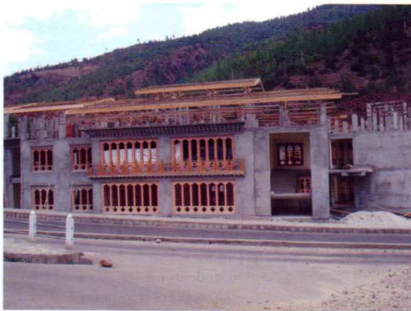
Tarayana Craft Centre under construction at Chubachu, Thimphu
