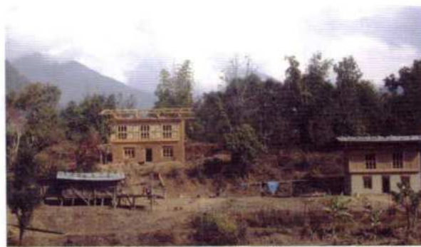
Improved Housing for the Olep Community
