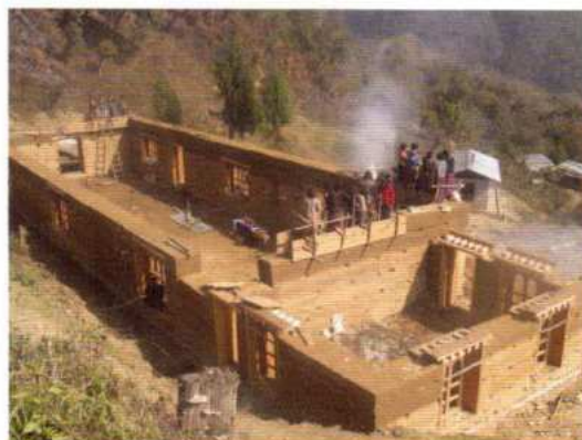
Construction of Girls Hostel at Sha Tasha Community Primary School
